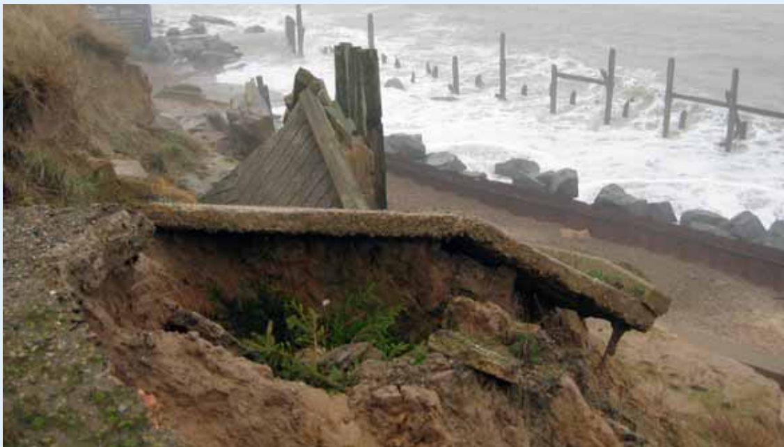
FIGURE 3-VII Evidence of cliff erosion at the site of the old lifeboat launch along the coast from Happisburgh 77
