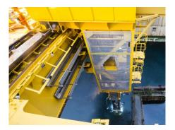
A key priority for Sellafield is dealing with the ageing FGMSP. This pond dates from the 1960s when it was built to store spent fuel from the Magnox stations. Over the years the pond has accumulated large quantities of waste material, including sludge from corroded fuel cladding, fuel fragments, skips and debris.
